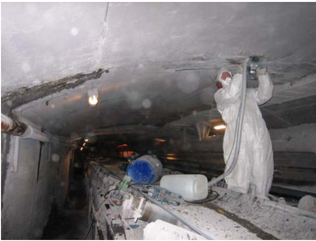
Tunneltak under utbedring.
